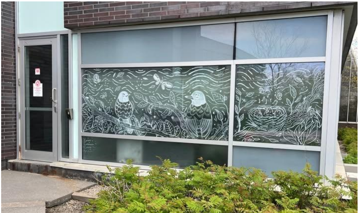
Window treatments at Carleton University help birds see glass and prevent window collisions. Photo by a Safe Wings volunteer.
